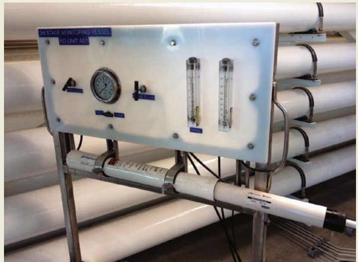
Figure 15 Third-stage monitoring system on RO concentrate.
