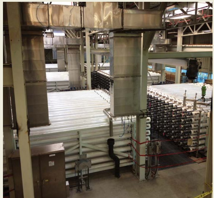
Figure 3 The GWRS expansion 30mgd capacity RO system.
