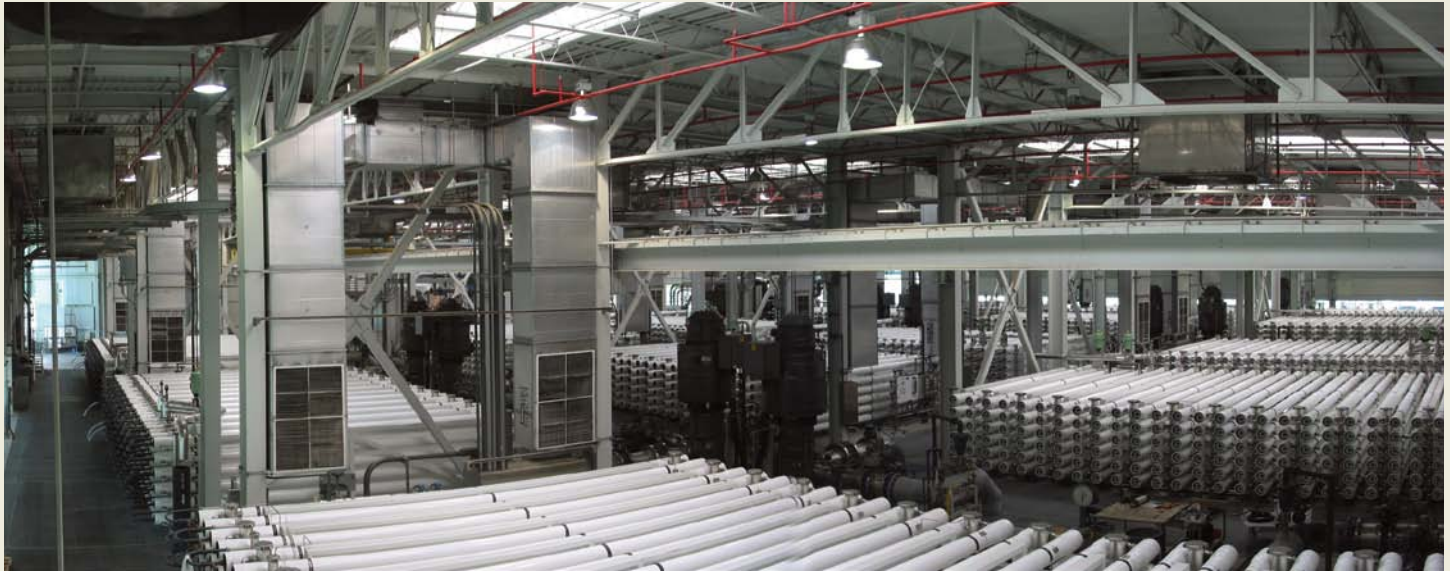
Figure 3 The GWRS expansion 30mgd capacity RO system.
