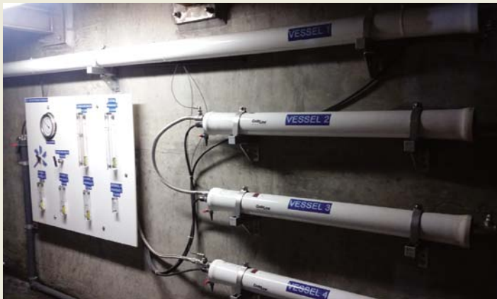
Figure 12 Third-stage monitoring system.
